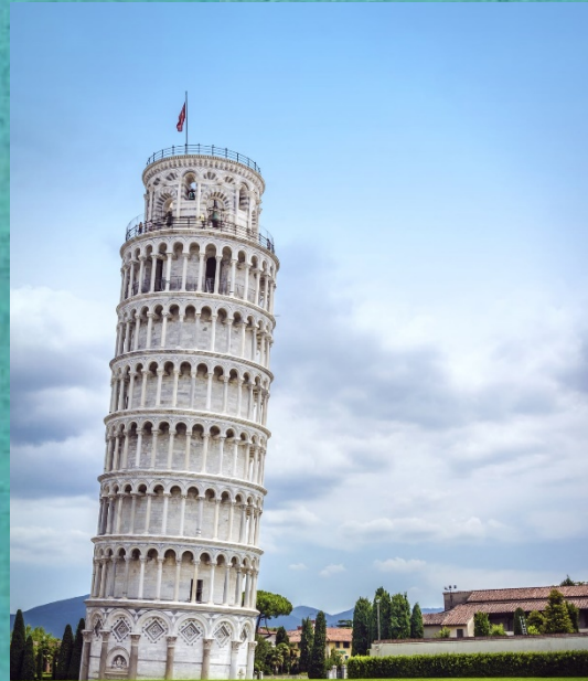
Leaning Tower of Pisa
