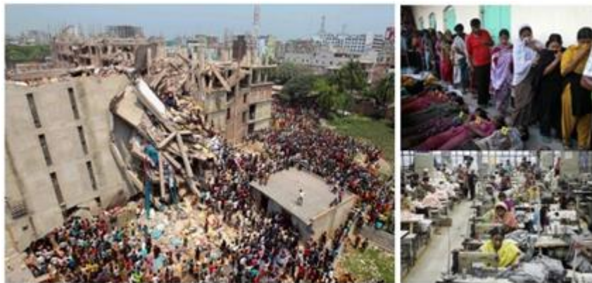
Dangerous working conditions
